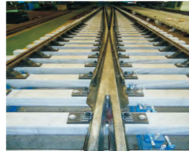
60kg/m Rail 1:18 Simple Turnout with Fixed Crossing
