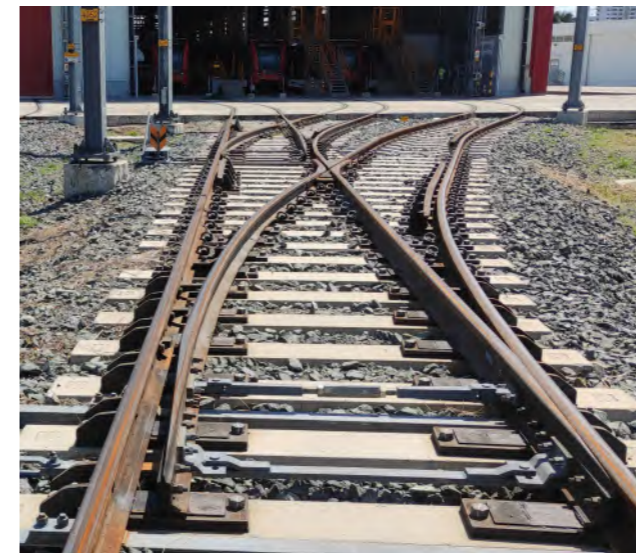
54E1 Rail 1:4 LRT Simple Turnout at Depot Exported to Philippines
