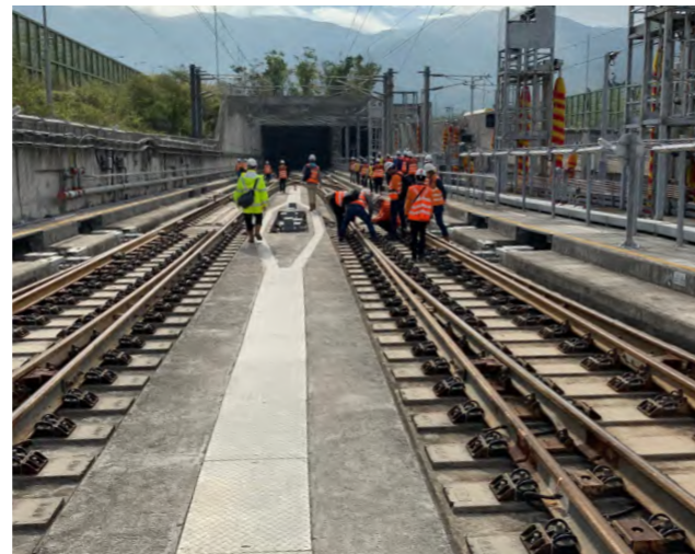
CHN60 1:12 High Speed Turnout for Guangzhou-Shenzhen-Hongkong PDL (Hongkong MTR)
