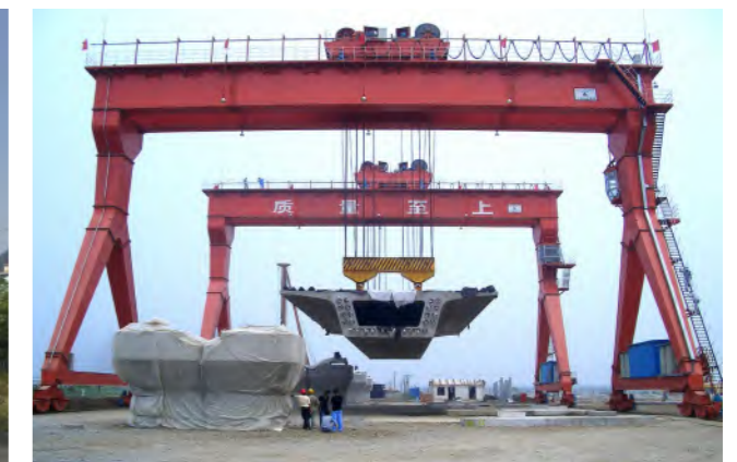
500 ton beam lifting machine
