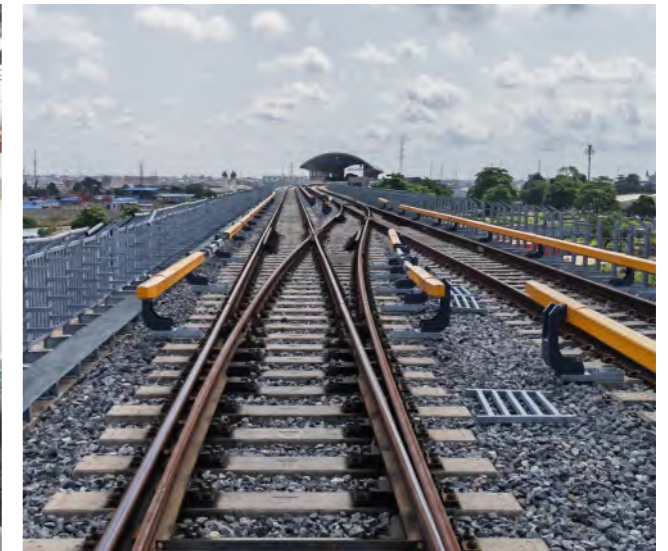
60E1 Rail 1:9 LRT Simple Turnout Exported to Nigeria
