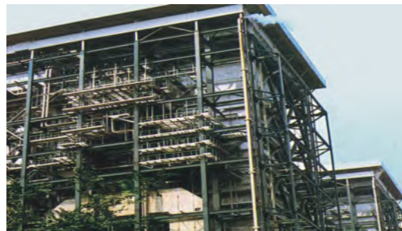
Power Generator Steel Structure Frames
