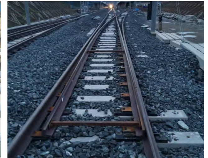
60kg/m Rail 1:12 Simple Turnout with Moveable Crossing Exported to Laos
