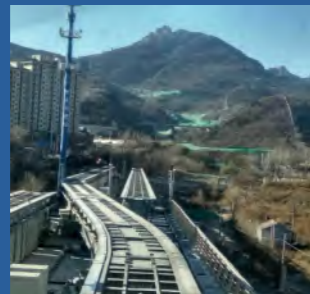
Medium and low speed maglev single crossover turnout
