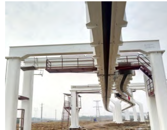
Turnout of Zhongtang Suspended Traffic System
