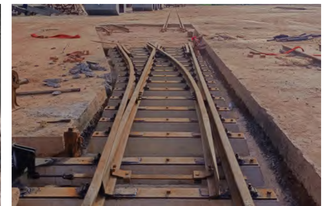
38kg/m Rail 1:4 Simple Turnout Exported to Laos
