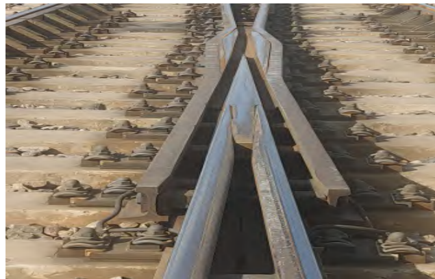
Forged High Manganese Steel Crossing
